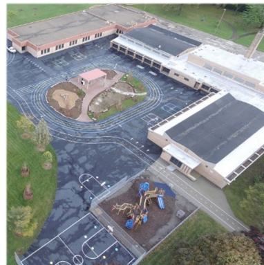
The Clement Avenue School (Milwaukee, Wisconsin) schoolyard redevelopment project can manage over 88,000 gallons of stormwater every time it rains. The school has removed approximately 22,000 square feet of asphalt and has replaced it with green and a mixed-use recreation and educational space.
